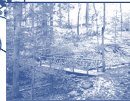
Upper Wooden Bridge
